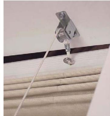
Figure 16 Attached Return Pulley
