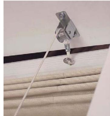
Figure 27 Attached Return Pulley
