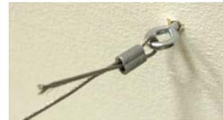
Figure 13 Guide Wire on Screw Eye
