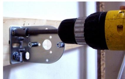
Figure 8 Fasten Motor Bracket
