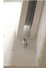
Figure 8 Screw Eye Fastened
