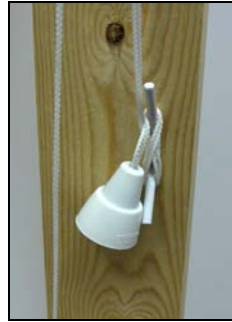
Figure 7 Cord on Cleat—Shade Down
