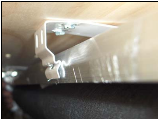
Figure 7 Cassette bracket unclipped
