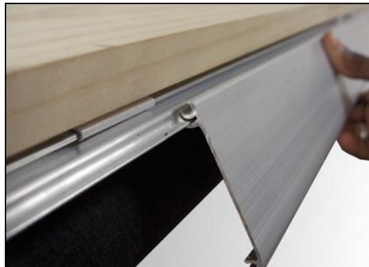
Figure 15 Align the groove on the cassette front with the top rail
