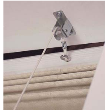
Figure 16 Attached Return Pulley
