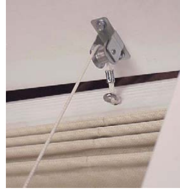
Figure 27 Attached Return Pulley
