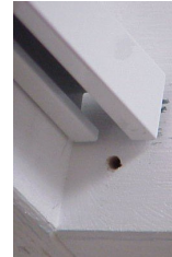
Figure 7 Screw Eye Hole Below Track
