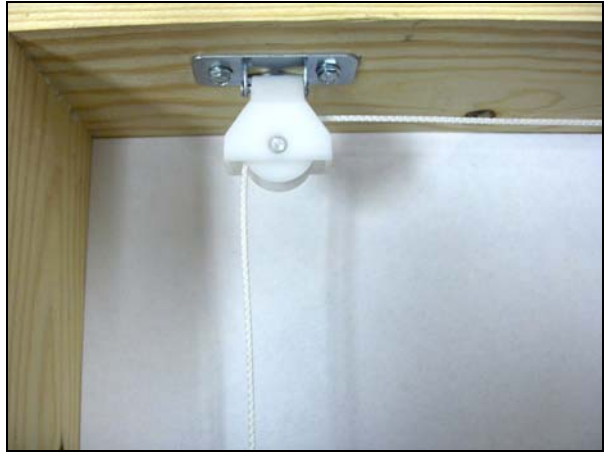
Figure 5 Pulley Installed
