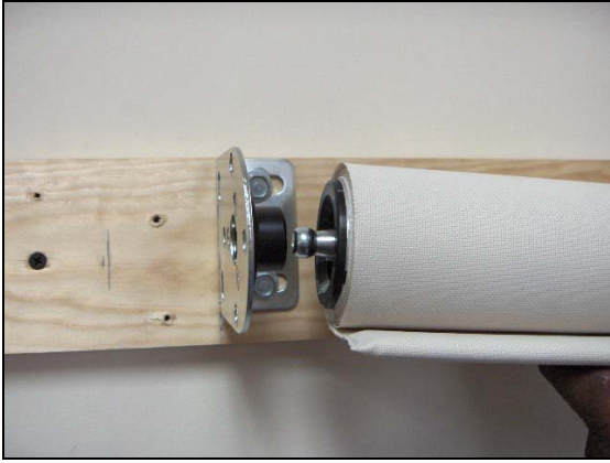
Figure 19 Motor Idler Going into Bracket
